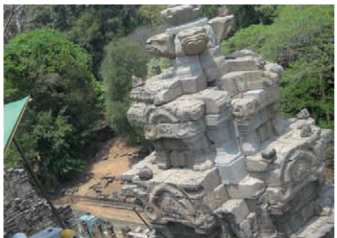
Work site of the French School of Asian Studies (EFEU): restoration of the Baphuon Temple in Angkor, Cambodia. © Éric Lamouroux.
