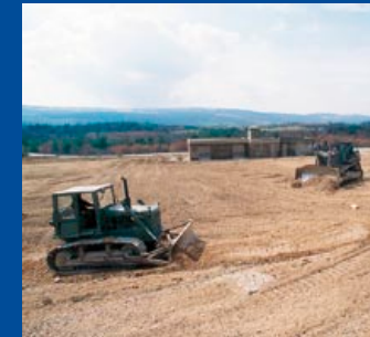
1998: dismantling is almost over
