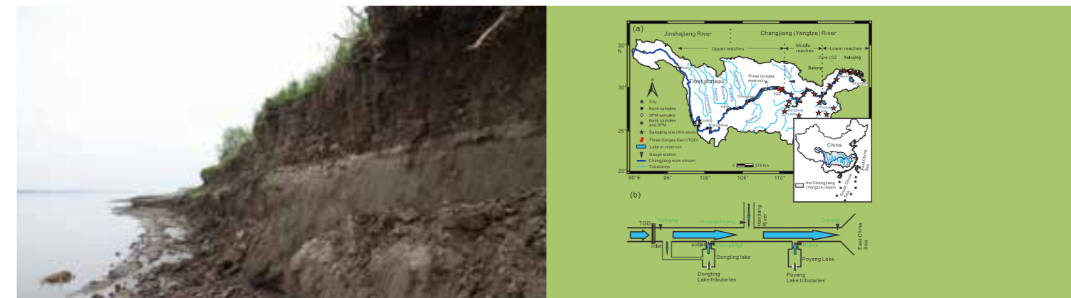
Strong river bank erosion downstream the TGD
