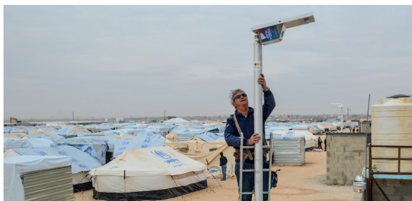
Installation of solar lamp posts in Al Za'atari refugee camp, 2012, Jordan
