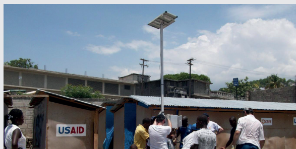
Installation of solar lamp posts, 2010, Haiti
