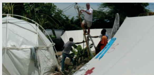
Installation of lamp posts in refugee camp, 2011, Horn of Africa
