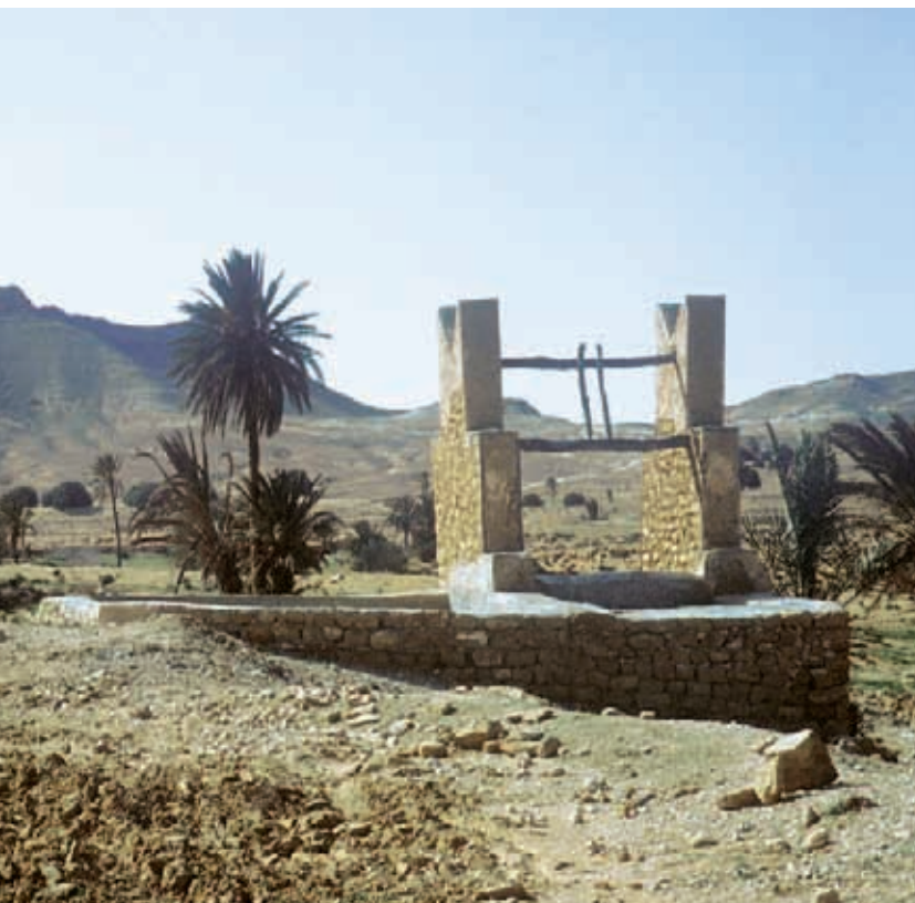
Traditional irrigation system (Tunisia) - © IRD/Jean Pouget
